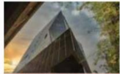
Chambers Project— The design firm came up with innovative solutions to make the most of the available space.
